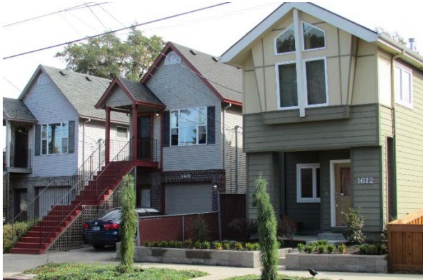
Houses with long runs of stairs supported by an above grade structure (middle) and ground entry (right)
